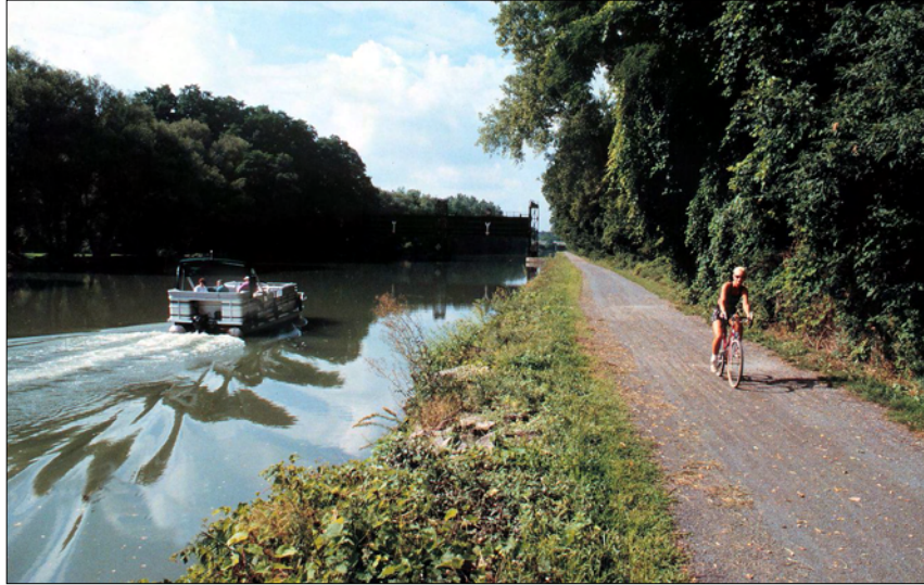
Figure 5-C – Limestone Dust Trail, 10'-wide Canalway Trail in Western NY
